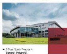
3 Tuas South Avenue 4 General Industrial
