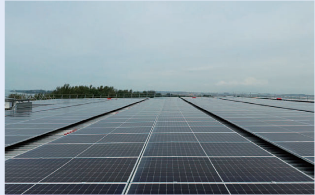
Newly installed photovoltaic panels at 51 Alps Avenue
