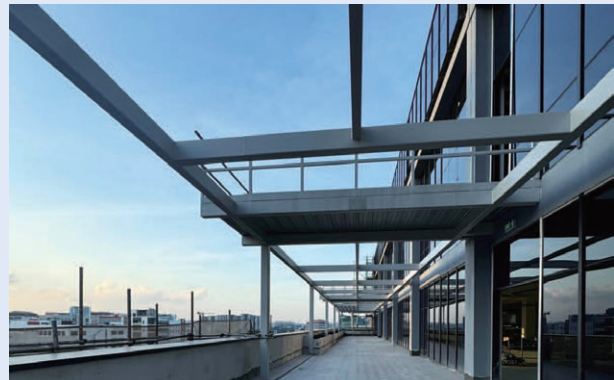
Low heat gain glass installed for new façade
