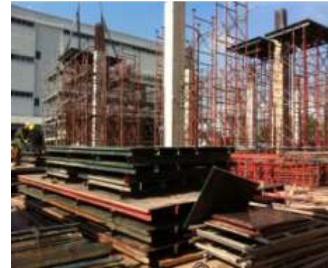
2 nd floor slab formwork in progress – Mar 12
