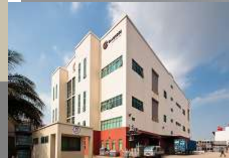
79 Tuas South St 5
