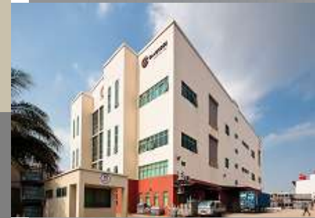
79 Tuas South St 5
