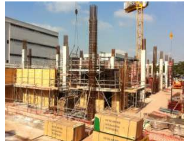
Casting in progress – Mar 12
