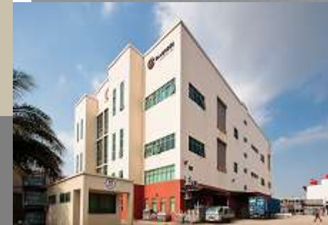
79 Tuas South St 5
