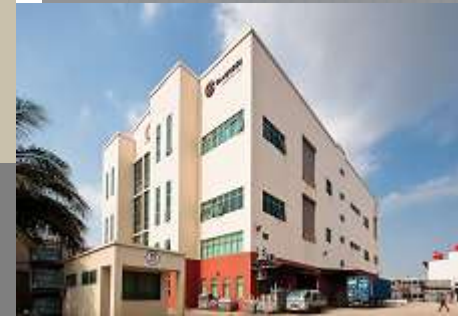
79 Tuas South St 5
