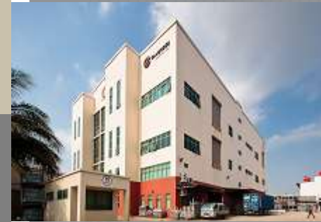
79 Tuas South St 5
