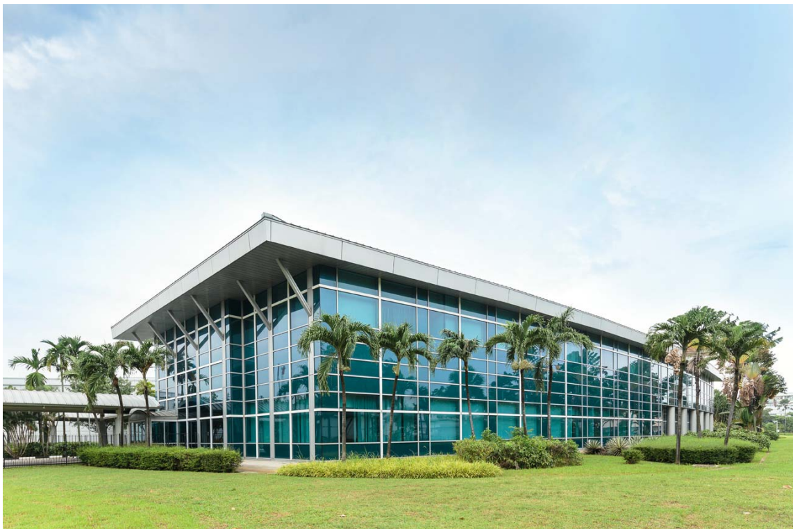
3 Tuas South Avenue 4
