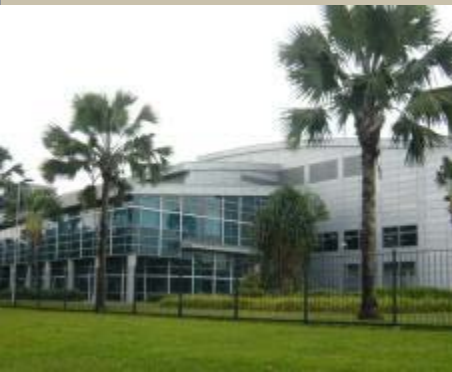
3 Tuas South Avenue 4
