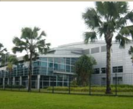
3 Tuas South Avenue 4
