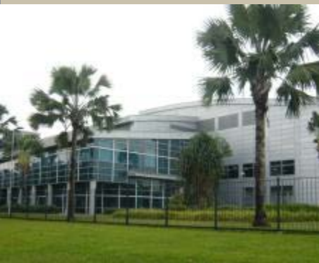
3 Tuas South Avenue 4
