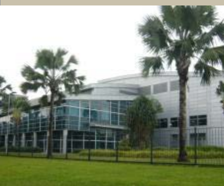
3 Tuas South Avenue 4
