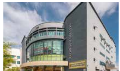
2 25 Changi South Avenue 2
