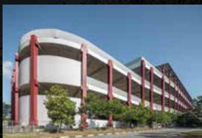
Acquisition of 15 Greenwich Drive
