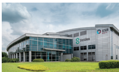
20 3 Tuas South Avenue 4
