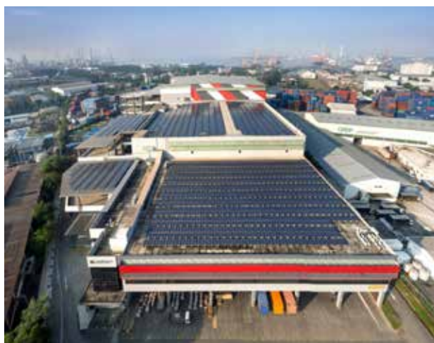
Solar panels on top of 3 Pioneer Sector 3
