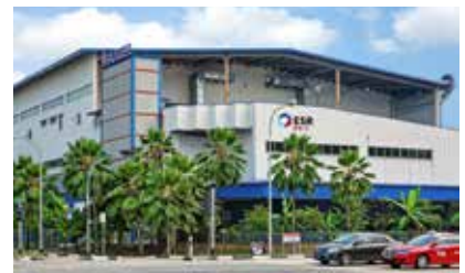
1 81 Tuas Bay Drive
