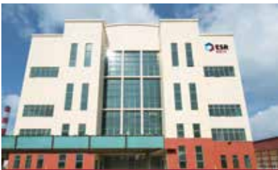
2 79 Tuas South Street 5
