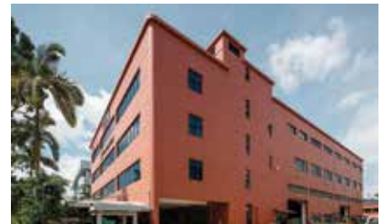
7 31 Changi South Avenue 2
