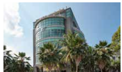
10 2 Tuas South Avenue 2
