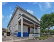
81 Tuas Bay Drive
