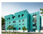
45 Changi South Avenue 2
