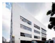
60 Tuas South Street 1
