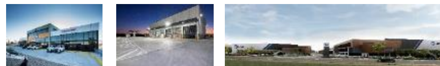
6 Skyline Crescent, 379 Sherbrooke Road, Bringelly NSW
