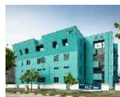
45 Changi South Avenue 2
