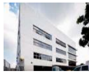
60 Tuas South Street 1
