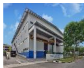
81 Tuas Bay Drive
