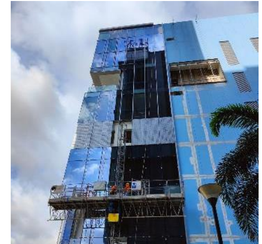
Building façade undergoing major facelift for a modern look
