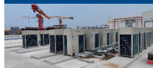
M&E enhancements in progress
