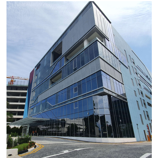
Building façade undergoing major facelift for a modern look
