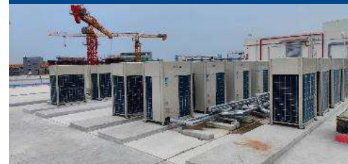
M&E enhancements in progress
