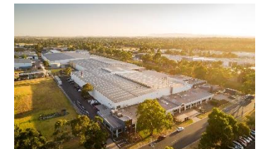
41-51 Mills Road, VIC
