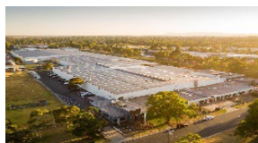
41-51 Mills Road, Braeside, VIC
