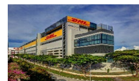
DHL Supply Chain Advanced Regional Centre
