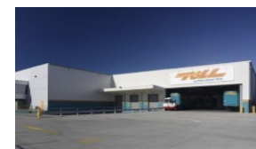
67-93 National Boulevard, Campbellfield, VIC
