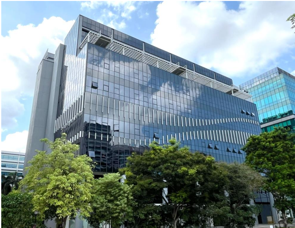
Completed AEI at 16 Tai Seng Street, Singapore
